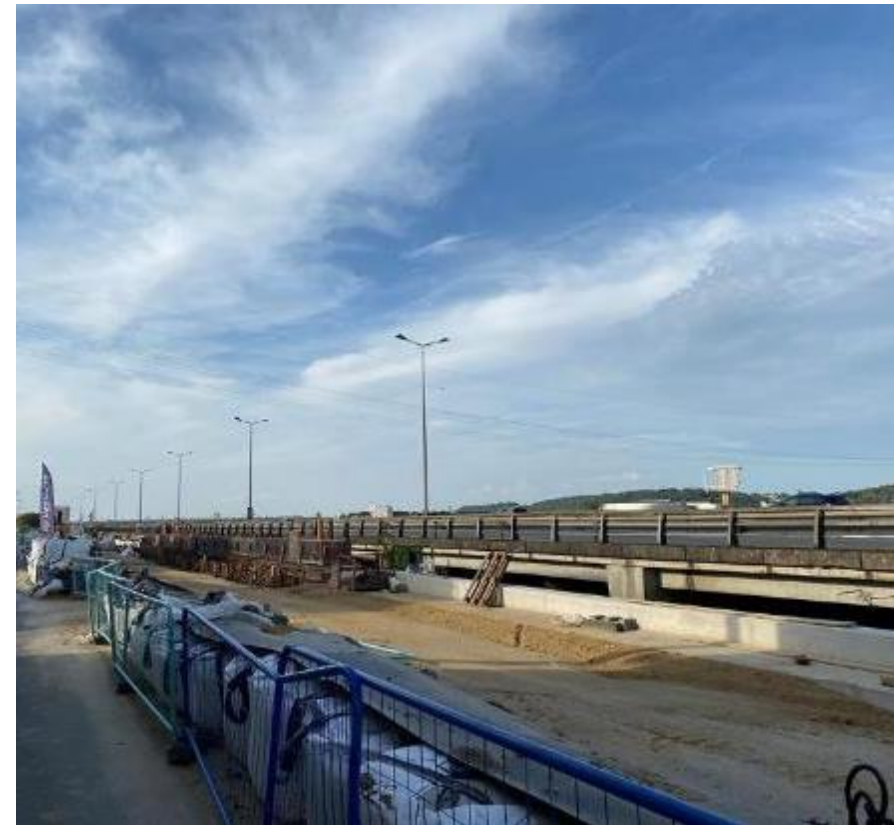
Consolidation digue quai Wilson 02/09/2024
